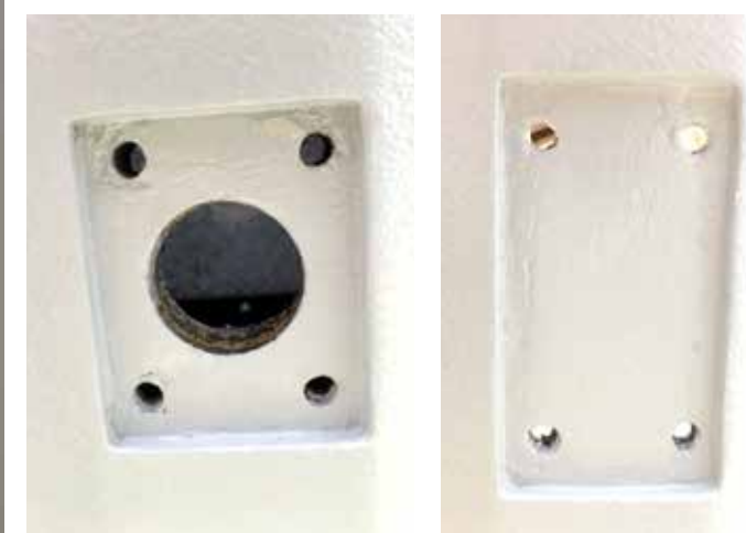
Rudder and strut area repair complete.
