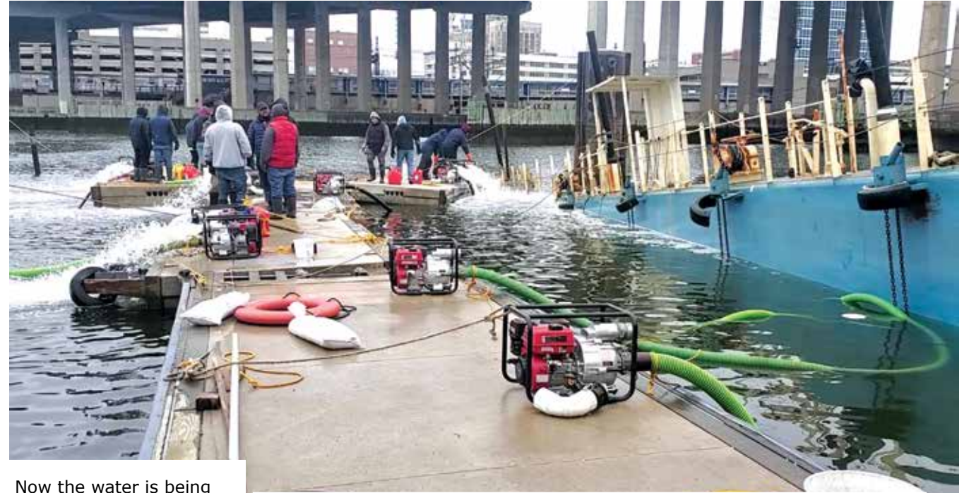
Now the water is being pumped out from the deck of the sunken dry dock. Air enters the compartments from above the water line to replace the weight of the water with air. Slowly buoyancy is being restored for the structure to rise.
