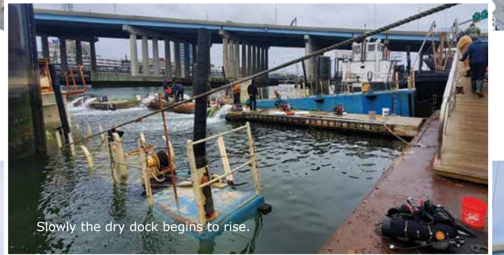
Now the water is being pumped out from the deck of the sunken dry dock. Air enters the compartments from above the water line to replace the weight of the water with air. Slowly buoyancy is being restored for the structure to rise.
