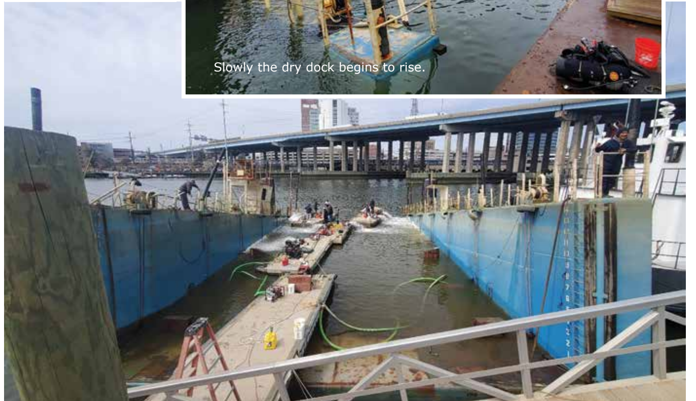
Now the water is being pumped out from the deck of the sunken dry dock. Air enters the compartments from above the water line to replace the weight of the water with air. Slowly buoyancy is being restored for the structure to rise.
