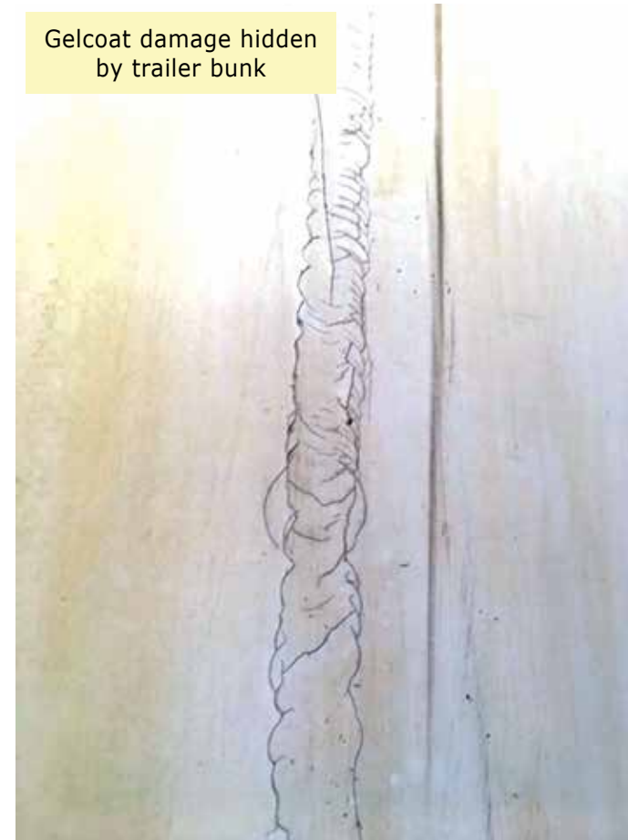
Fiberglass cracks hidden by trailer bunk
