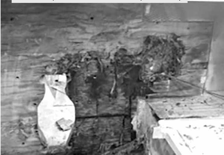
Transom replacement is a common repair necessity.
